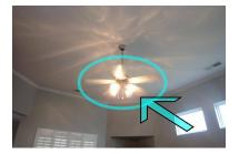
7. The glass portion of the light fixture located in the following areas was noted to be cracked/broken at the time of the inspection. Replacement is advised to insure safety and proper operation of the fixture.
